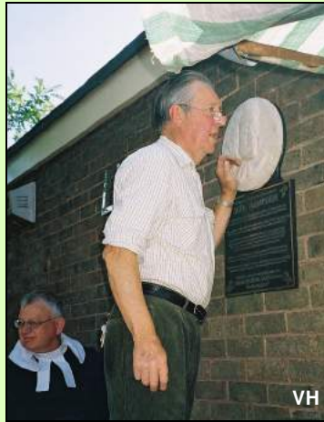
Waiting for the adhesive to set, while Sam Hearn holds the ladder
